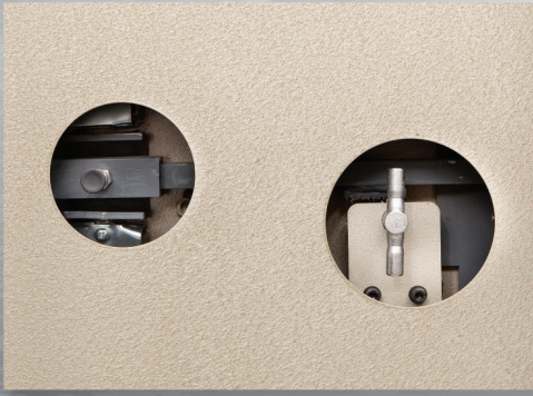
Internal Emergency Door Release
